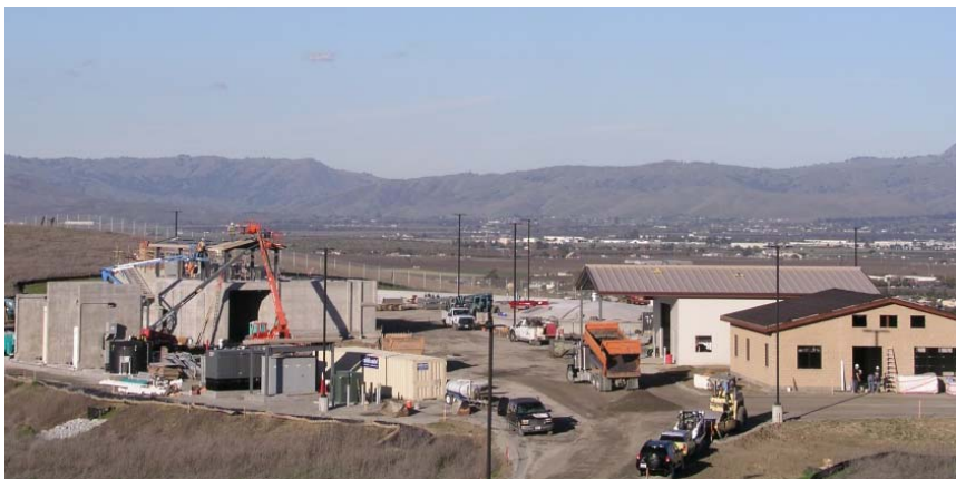
Figure 2-6. West Hills Water Treatment Plant
