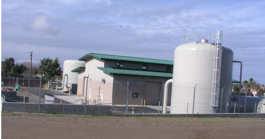
Figure 2-5. Lessalt Water Treatment Plant
