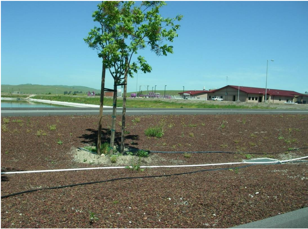
City Water Reclamation Facility
